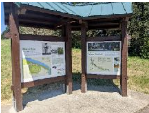
Painted over graffiti at kiosk
